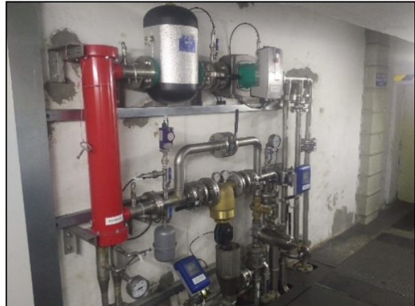
Fig 22 - Bearing & Seal Water Filtration System
