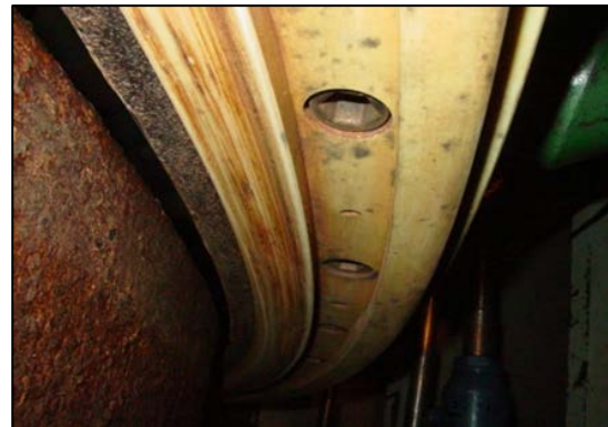
Fig 15 - Sealing Face - 1 year Inspection
